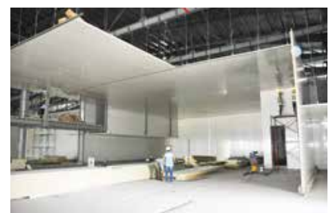
Project under construction
