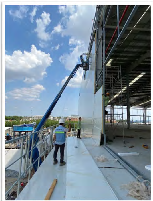
Supply & Erect Factory External Panel
