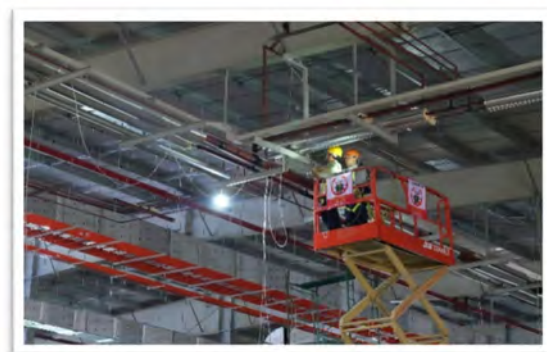
Install Refrigeration System Piping
