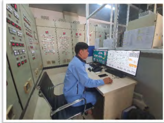
SCADA for Refrigeration System
