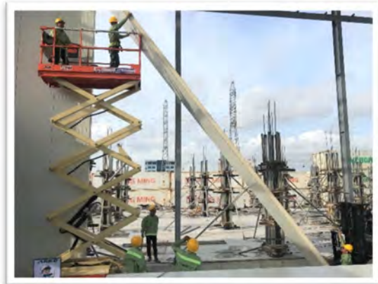
Erecting Cold Warehouse Wall
