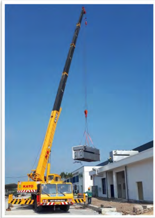
Lift-up & Installation Condenser
