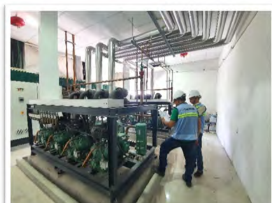
Install Freon Refrigeration System
