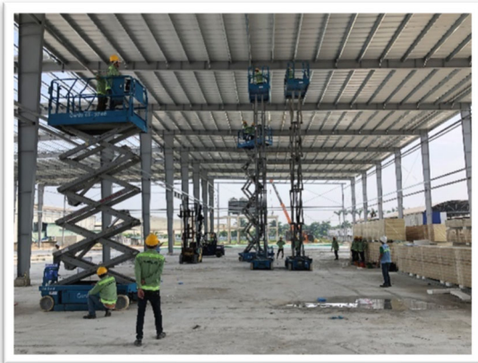
Erecting Cold Warehouse
