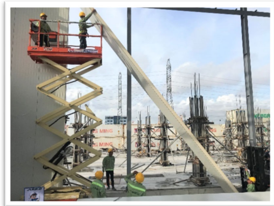
Erecting Cold Warehouse Wall
