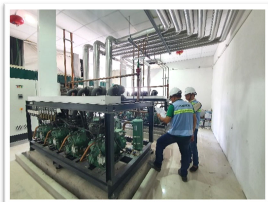
Install Freon Refrigeration System
