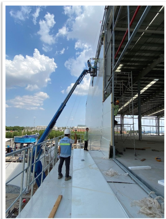
Supply & Erect Factory External Panel
