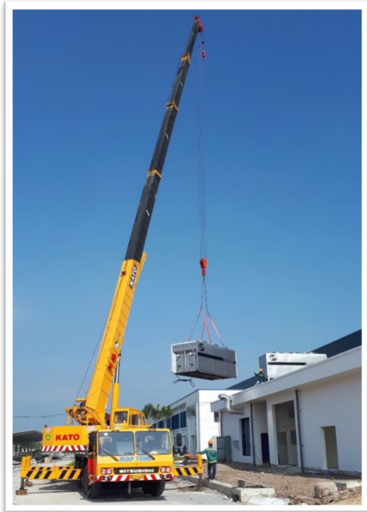
Lift-up & Installation Condenser
