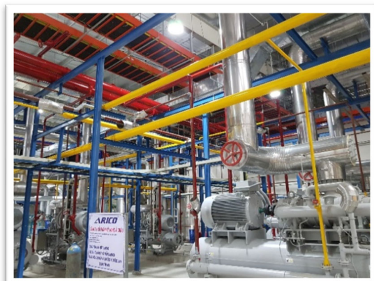
Install NH 3 Refrigeration System
