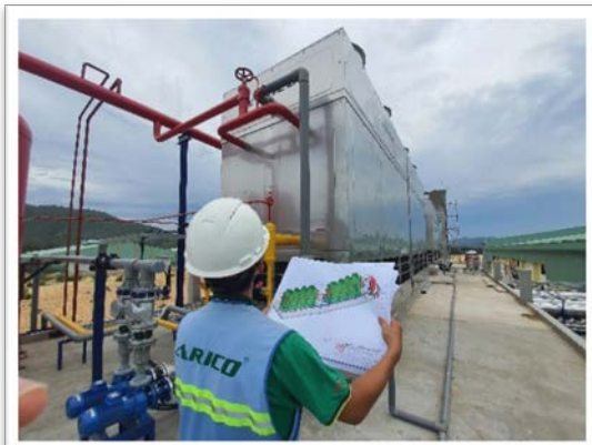
Inspection Stainless Steel Condenser
