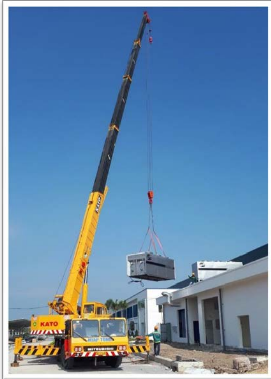
Lift-up & Installation Condenser
