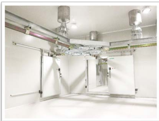
Supply & Erect Doors & Railway System
