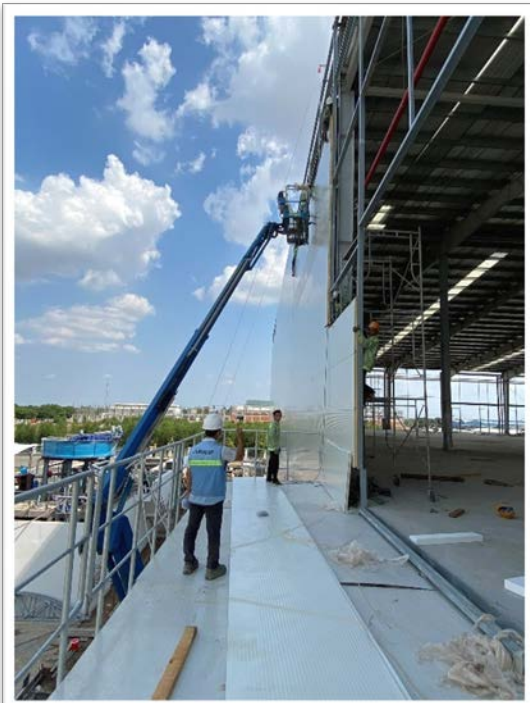
Supply & Erect Factory External Panel
