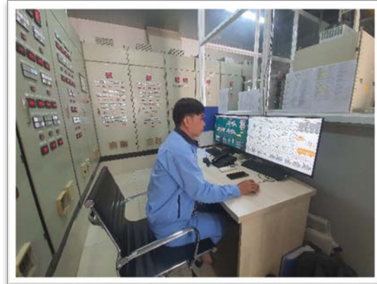
SCADA for Refrigeration System
