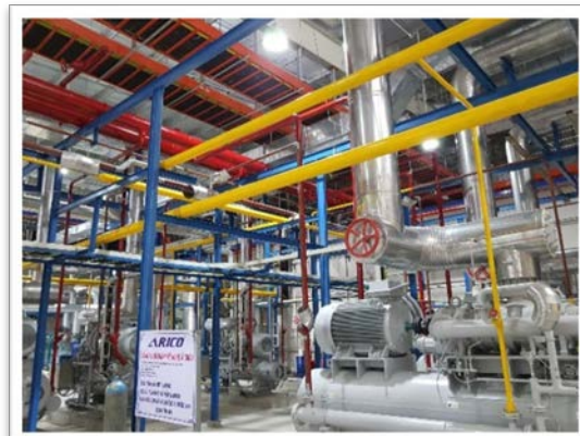
Install NH3 Refrigeration System
