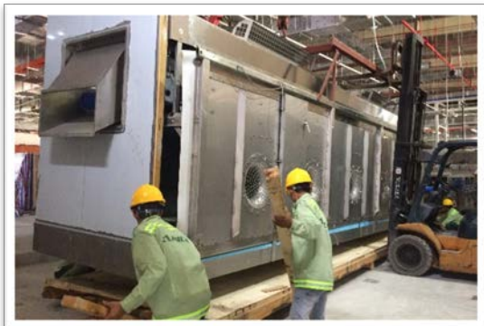
Supply & Install IQF for Fruit
