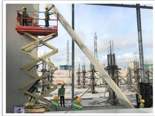
Erecting Cold Warehouse Wall
