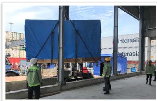
Unload & Prepare for Erection
