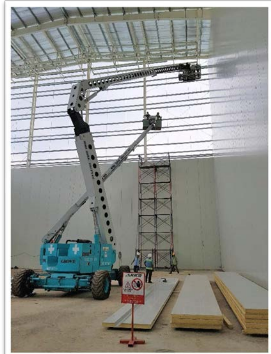
Supply & Erect ASRS Cold Storage
