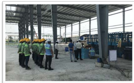
Prepare for Breaking Ground
