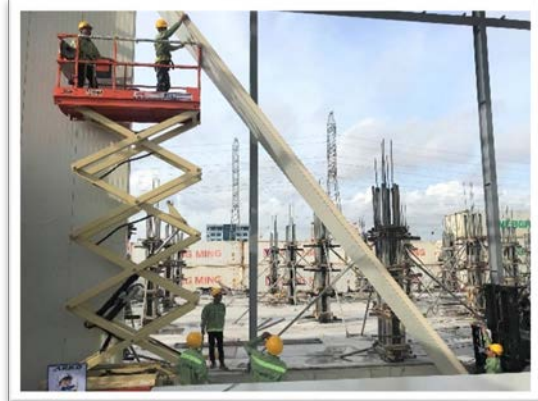
Erecting Cold Warehouse Wall
