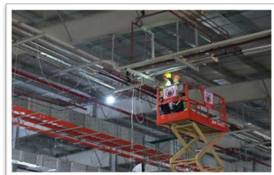
Install Refrigeration System Piping
