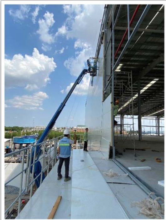
Supply & Erect Factory External Panel
