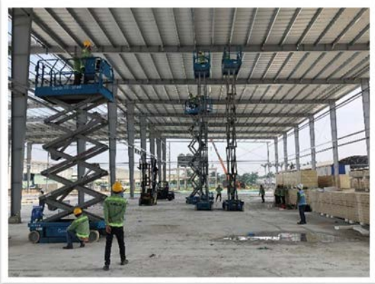
Erecting Cold Warehouse
