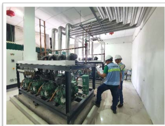
Install Freon Refrigeration System
